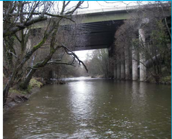
Figure 1-3 A55 Road Bridge
