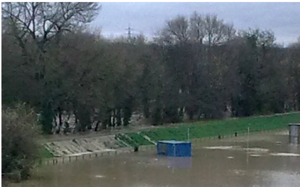
Figure 4-7 Overtopping of left Elwy embankment to Cattle Market
