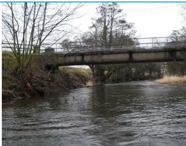
Figure 1-4 Sewage Works Bridge
