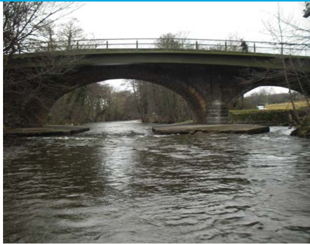
Figure 1-2 St Asaph Old Bridge (all of bridge not shown)
