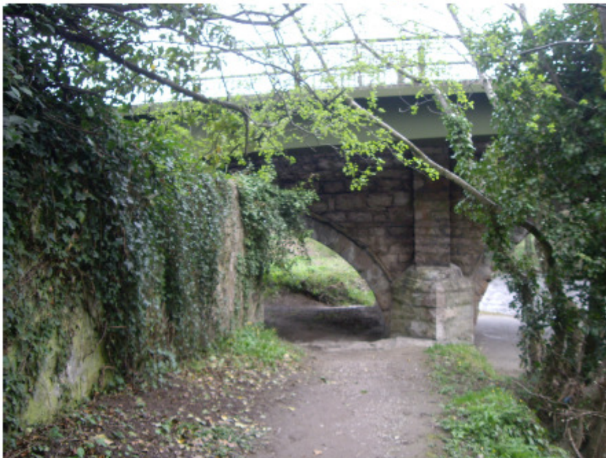
Figure 3-2 St Asaph Old Bridge and wall upstream
