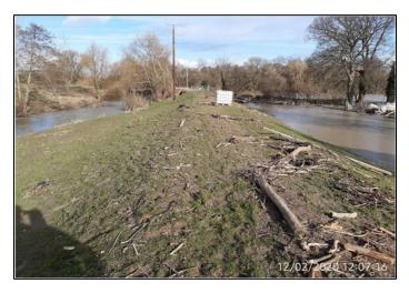
Figure 38: Wrack & debris deposits showing line of overtopping (NRW, 2020)
