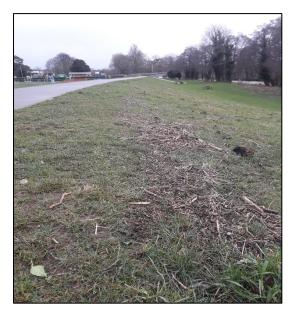
Figure 108: Wrack mark common emb (NRW, 2020)
