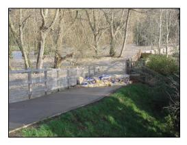
Figure 91: River gravel deposit on Foxons Ramp (NRW, 2020)
