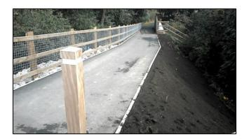
Post-event topographic survey completed by NRW confirmed that the as-built levels for Elwy left bank Roe Parc defences were within engineering tolerances for hard and soft defences (Figure 26).
